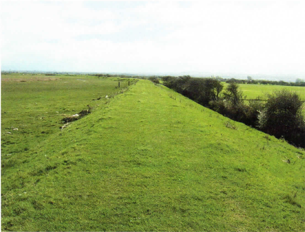
Plate 9. Clwyd Embankments at Clwyd PS looking south east towards Rhuddlan
