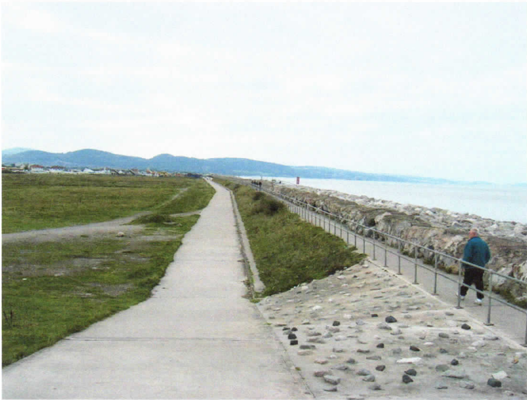
Plate 5. Landward face of new Towyn Defence (Section B)
